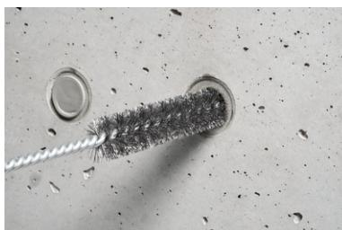
Soiled distance tubes must be thoroughly cleaned before installing the **STOPPER**.
