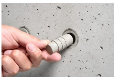
Whether using cones or lip seals, the **STOPPER in** can be used as the outer closure of the distance tube.
