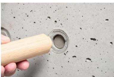
Whether using cones or lip seals, as the outer closure of the distance tube, the **STOPPER in** can be driven in until it is recessed.
