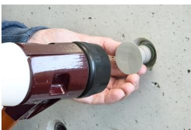
The **STOPPER maxi** is installed by driving it in with a hard rubber mallet (weight 1500 - 2000 g) using reasonable force.
