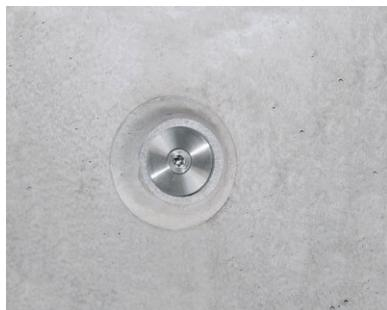
**STOPPER SCREW type covered** mounted in tie point with cone.
