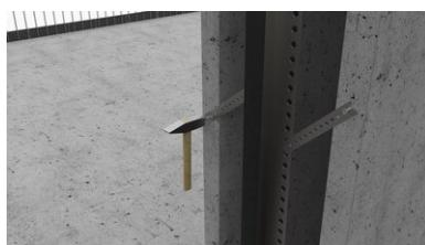
The mounting bracket is fixed with a drive-in plug.
