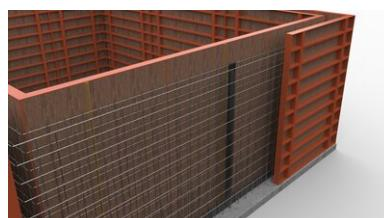
The **SFG profile** is set vertically and overlapped with the joint sheet metal (overlap  $\geq 5$  cm).
