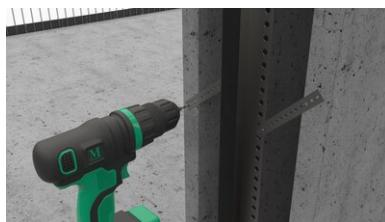
The wall formwork is drilled in order to fix the mounting bracket.
