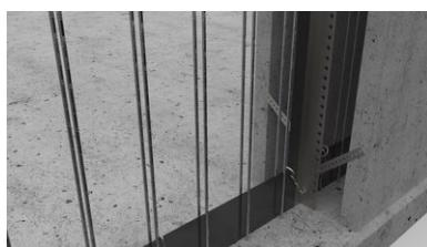
The overlapping area on the floor/wall joint sheet metal is secured with two fixing clips.
