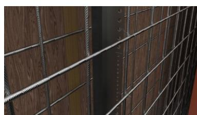
Use the foldable, perforated retaining plates to fix the **SRF profile** to the reinforcement.
