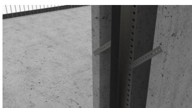
The adjustable mounting brackets are adjusted to fix them on the face of the cavity wall.
