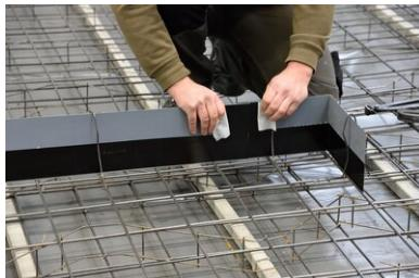
Overlap the **VB JGS joint sheet metal** by at least 6 cm and press the two ends firmly together.
