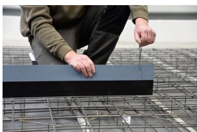
Place the **VB JGS joint sheet metal** in the centre of the rising wall on top of the upper reinforcement layer.
