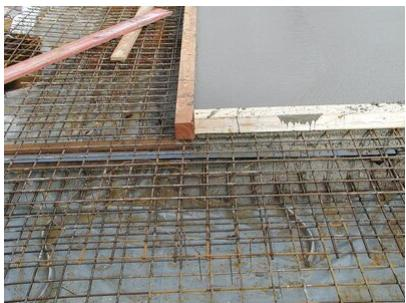
In the second concrete segment, as soon as the protective foil has been removed immediately before concreting, concrete can be placed directly against the stopen panel joint sheet metal ABS.
