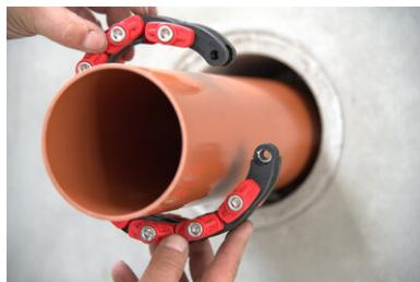
When using a **MASTER-SEAL** modular seal in combination with an existing installation, the "open" modular seal is placed around the existing medium pipe and closed as described at the beginning.
