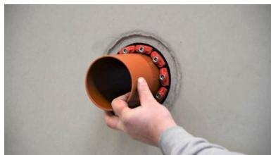
Push the **MASTER-SEAL** modular seal over the medium pipe, insert both into the preserved core drill hole and position the **MASTER-SEAL** modular seal appropriately. The **MASTER-SEAL** modular seal must be installed as close as possible to the outside of the wall ( earth-side, water-side).
