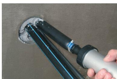
Fill the duct completely with **FLEX 2000**.
