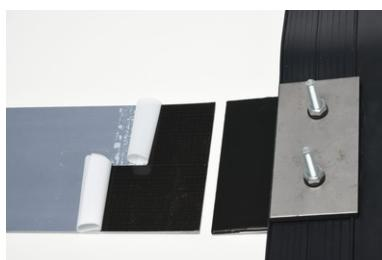
The protective foil of the joint sheet metal to be connected must also be removed.
