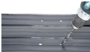
At the marked position, holes with a diameter of 10 mm are drilled into the joint tape.
