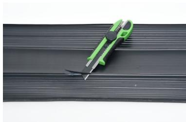
Within the marked area, the water barriers or edge anchors are removed with a sharp knife.
