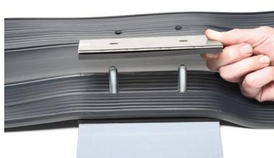
Lay the steel plates, the intermediate plates and the joint tape on top of each other as shown in the picture and the sketch below and join them together with the screws.
