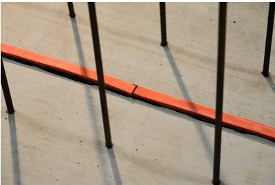
Straight butt joint
